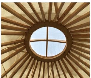
On our 20-foot Yurts we use kiln dried dimensional lumber for extra strength over the larger spans. (Natural poles can be used on the 20-foot yurt with special request)
